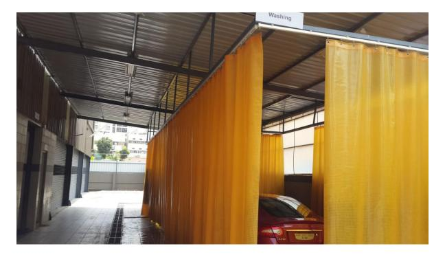
• MS powder coated , frame reinforced to the ceiling. Attached to the frame is a aluminum fixture and Rollers and S hooks for easy movement and convenience of folding the curtain and cleaning them.
