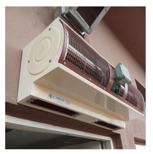
A high end and state-of-the art laboratory and research center needed a sophisticated Air Curtain at the entrance to prevent loss of pressure.
