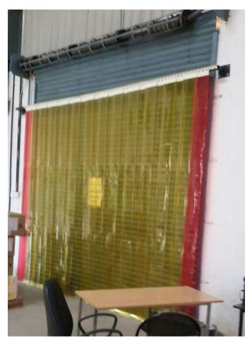
•MS Support provided at a lower height from the actual opening to economize use of materiel with the RED colored PVC to indicate the overall opening. Typically installed in Food industry.
