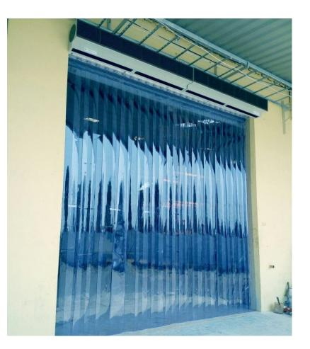
• PVC Strip Curtain and Air Curtain typically installed in heavy shuttered area which has frequent movement of men and materiel and to avoid escape of conditioned air, entry of insects and dust. This is a part of GMP specifications.
