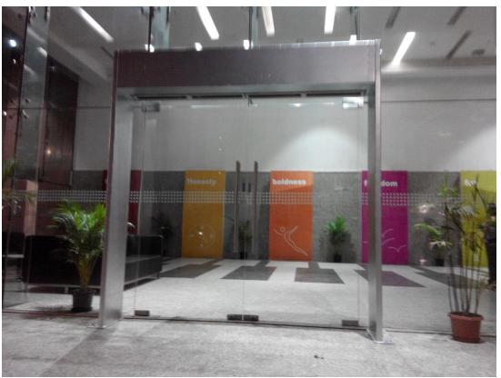
•Air curtain encased in Stainless steel structure and grouted to the floor to blend with the décor and aesthetics of the facility.
