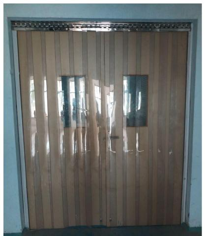
•In a typical Pharma and food processing industry, to avoid contamination, odour and micro dust, PVC Strip curtains are reinforced along with Hermetically sealed doors.
