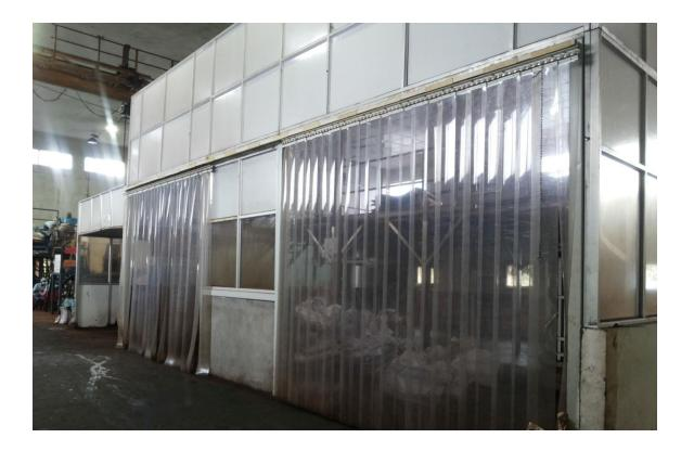
• PVC Strip curtain sliding door of height 12 ft. Fixed on aluminum railing with rollers to enable sliding for movement of raw materiel and allows flexibility of movement of men with ease.
