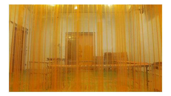
•Effectively installed in a large shop floor for materiel movement which are sparingly opened while movement of people is through a separate entrance . Both protected by PVC Strip Curtains to maintain a clean environment
