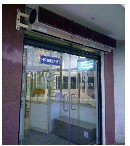
•In locations where the entrance does not provide for mounting the air curtain, we provide for additional fabrication so that it can be supported and reinforced according to the site requirements
