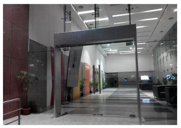
•Air curtain encased in Mild steel, painted silver color and grouted to the floor to blend with the décor and aesthetics of the facility.
